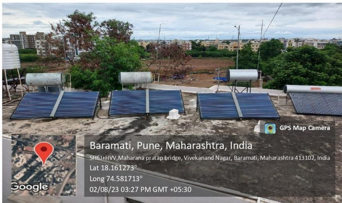
Solar Heater at Rooftop of 'D' Wing of Girl's Hostel
